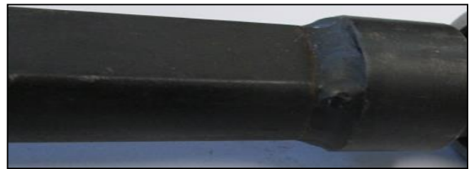
Figure 35: Welded shaft connection on 'Wysco' column
